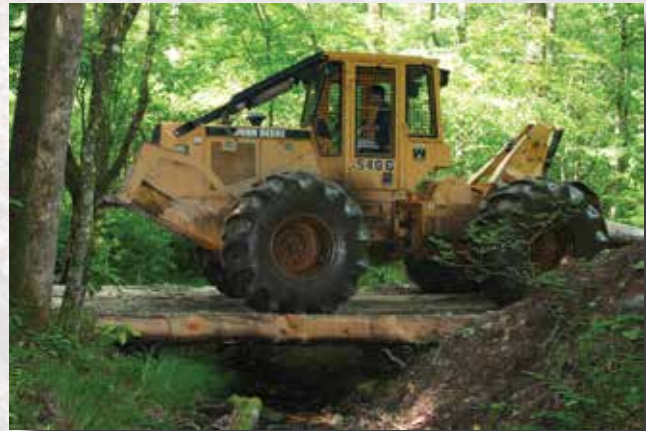
Figure 1. A skidder bridge that is temporary and will be removed after logging.
