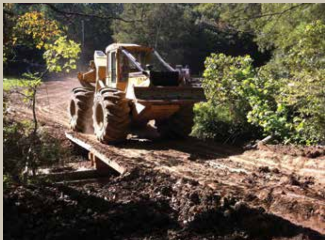
Figure 4. Wooden mats used to form a temporary elevated stream crossing for skidding logs in south-central Kentucky.
