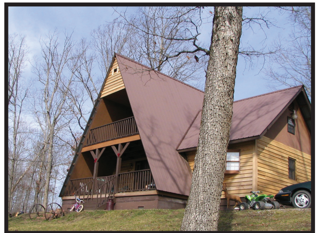
Homes with nonflammable roofs such as this metal one are more likely to survive a wildfire than those without defensible space and flammable roofs.
