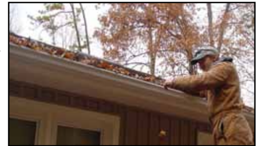
Simple tasks such as keeping your gutters free of debris can help make your home more Firewise by reducing the likelihood that a burning ember will start a fire in your gutters.
