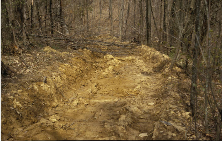
Figure 2. Under the new BMP requirements ruts like this may or may not be required to be fixed depending on whether or not they are causing a water quality problem or not.
