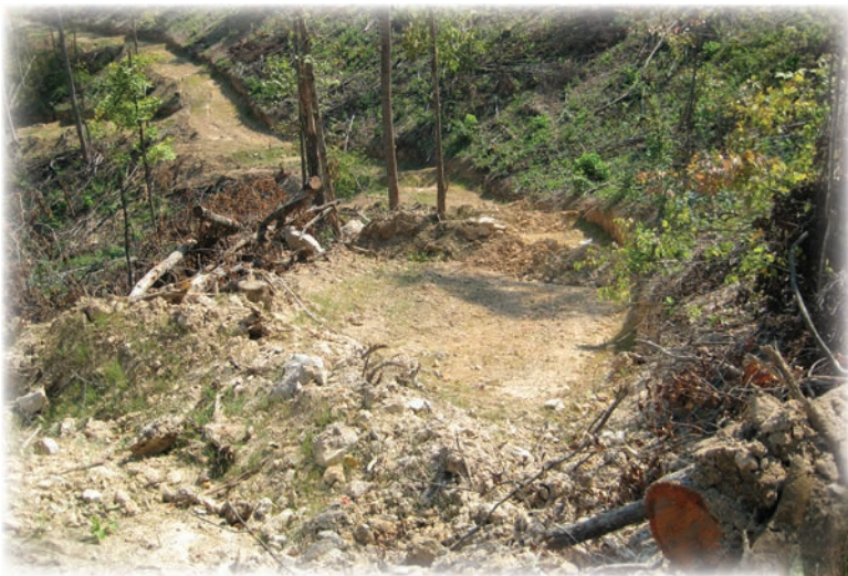
Figure 1 (above): When skid trails are no longer in use any ruts should be removed and permanent water control structures such as water bars installed. Skid trails that are erodible should be seeded to initiate grass cover.
