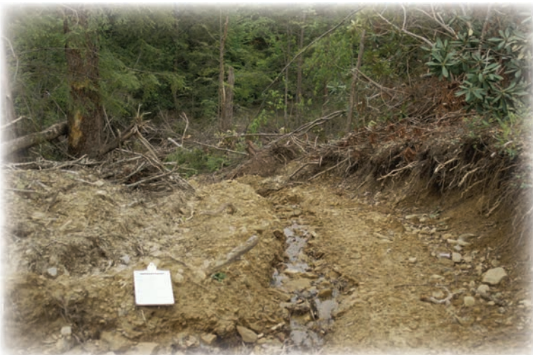
Figure 3. When BMPs are not used rutting of skid trails and haul roads can occur (above) or mud holes around streams and channels are common (below).
