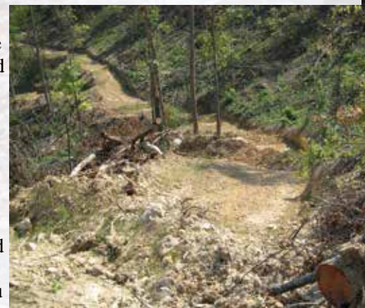
Figure 2. Typical water bars constructed by loggers. They work efficiently to control water but are not passable.
