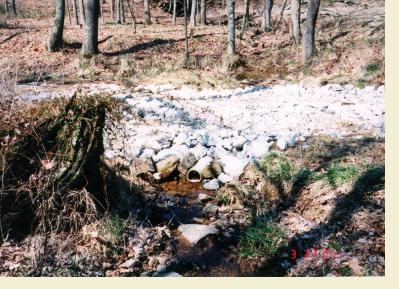
**Protecting Water:** Protecting water is a critical part of sustainable management. Here rock and a PVC pipe are used to cross a small woodlands stream in western Kentucky.
