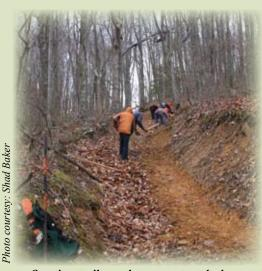
Overtime trails can become entrenched and require maintenance. In addition to rehabbing the trail surface, working to redirect water off the trail (by busting through the berm on the left and installing cross-drain structures) can increase the life of the trail. Try to include users in the maintenance and upkeep of the trail as it is their best interest that the trail be kept in peak condition.
